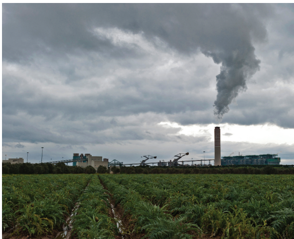
BRINDISI POWER PLANT. © Ida Santoro
