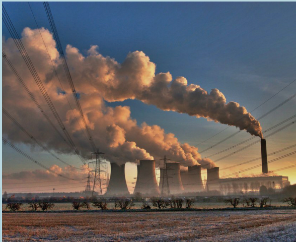
EGGBOROUGH POWER PLANT. © John Mabbitt
