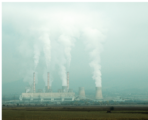
AGRIOS DIMITRIOS POWER PLANT. © Ioannis Tokaris
