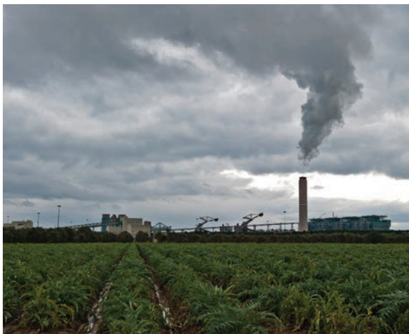
BRINDISI POWER PLANT. © Ida Santoro
