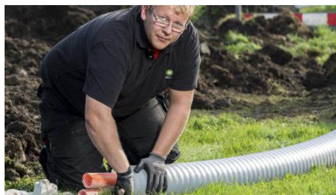
Installing a local district heat network in Germany. Source: AEE/Langrock
