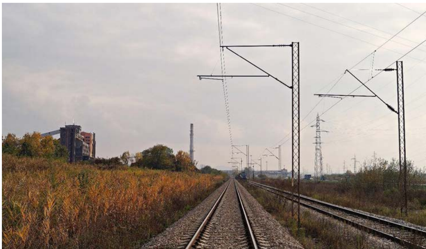
Image 21: The industrial railway connecting the Kolubara mining basins with the TENT in Obrenovac
