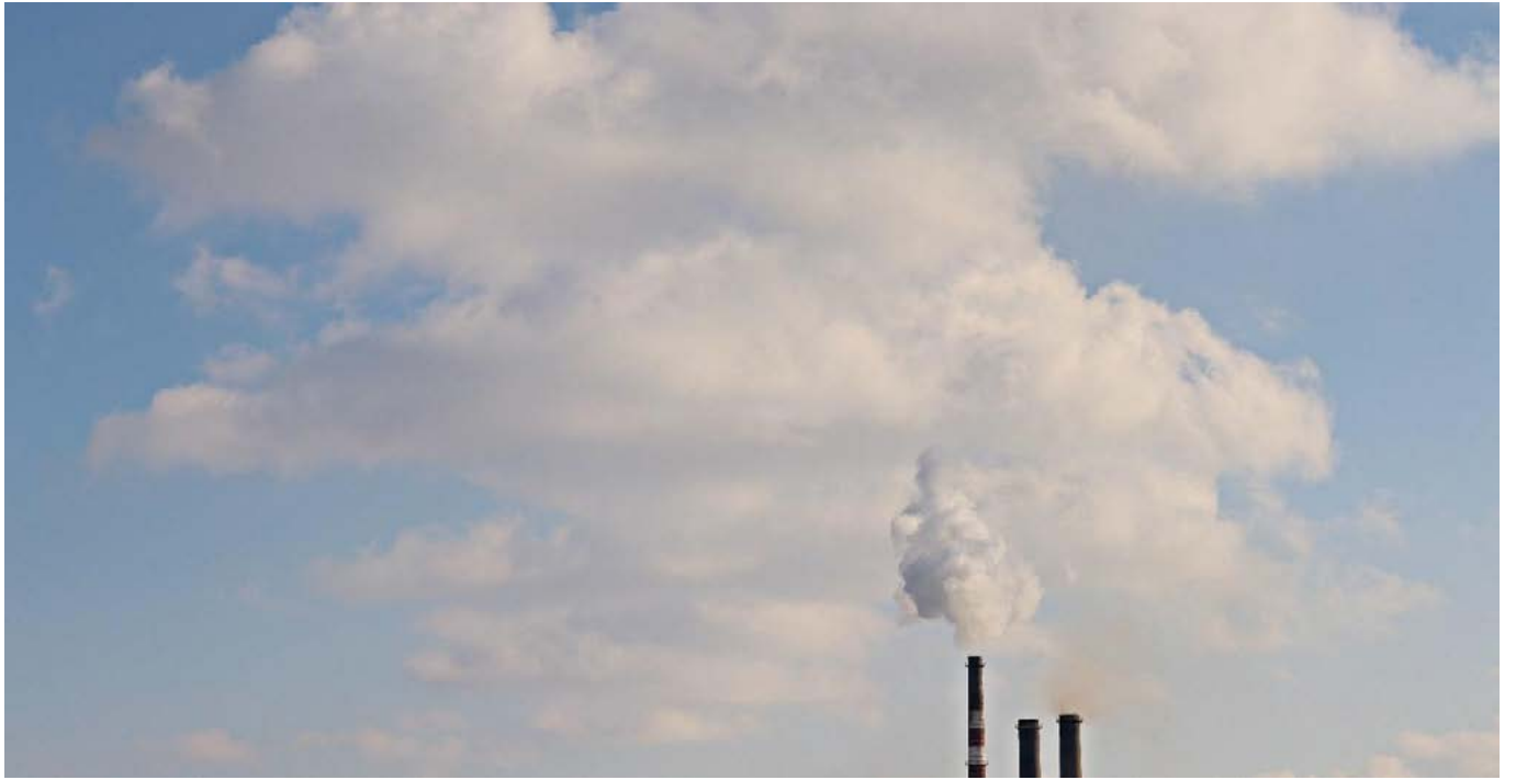
Image 6: The chimneys of TE Kolubara as seen from the Ibar Highway
